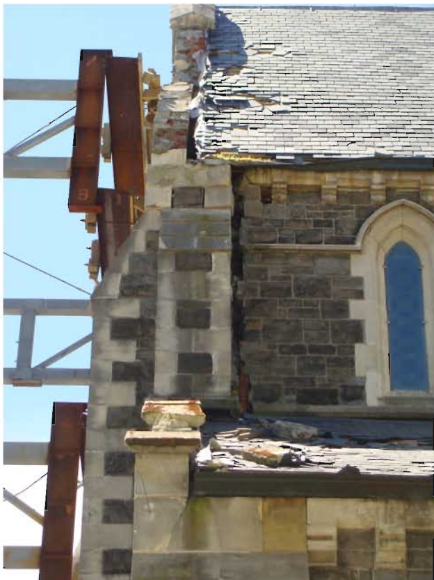
SW corner junction 3 rd November
