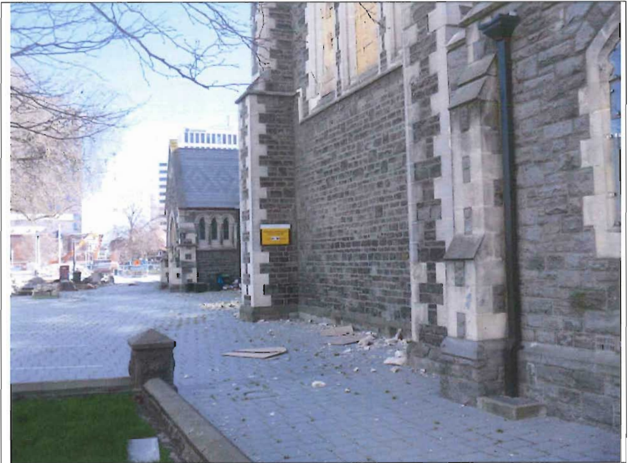
Photograph D – General view of south side of Cathedral showing no liquefaction or ground settlement damage
