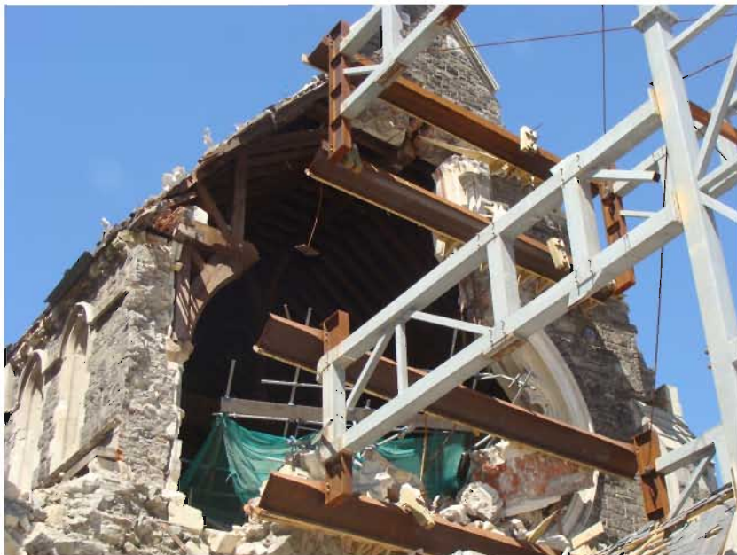
West wall 3 rd November
