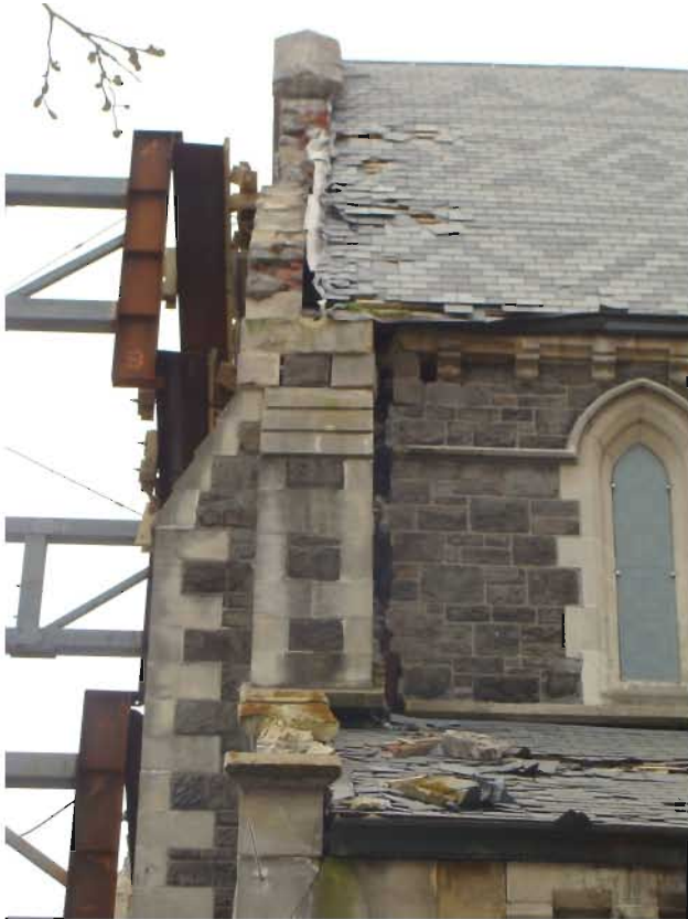
SW corner junction 22 nd September
